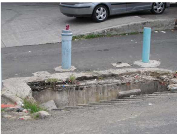
Above: Typical examples of current condition of Kerb Inlets
