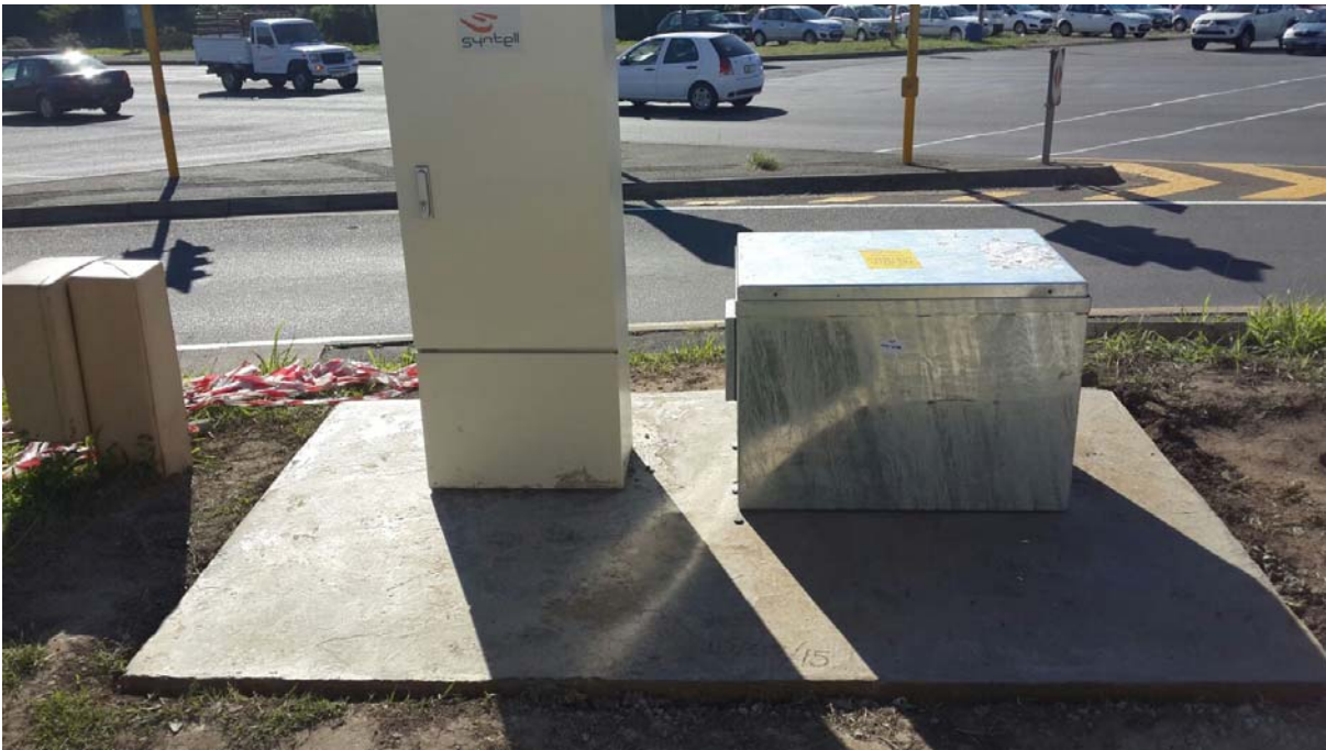
Figure – Installation of UPS equipment to power traffic signal equipment
