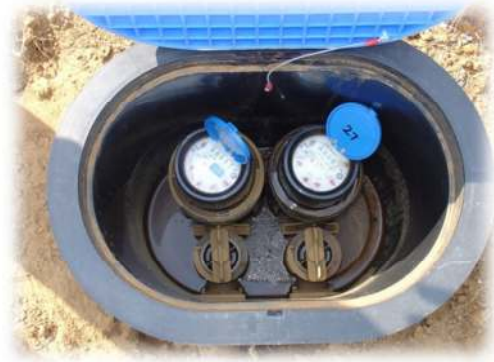
Double meter box considered as two connections
