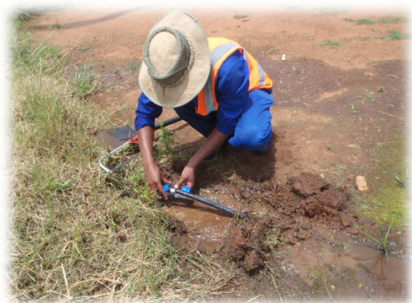
Repairing leaks will reduce physical losses
