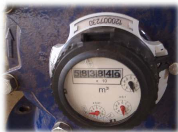
Excluding the x10 factor on bulk meters increases commercial losses (Meter reading = 583849 x 10 = 5838490)
