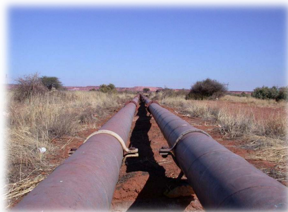
Long sections of transmission mains should be excluded from the length of reticulation
